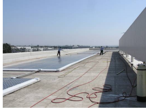
Figure 4: Array washing crew
