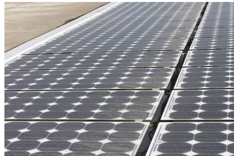
Figure 5: Modules prior to cleaning
